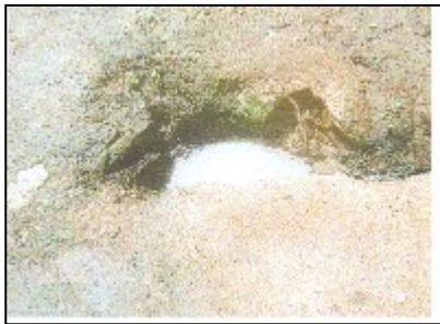
Figure 1: Miniature manhole not drained
