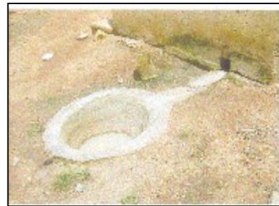
Figure 2: Uncovered miniature manhole
