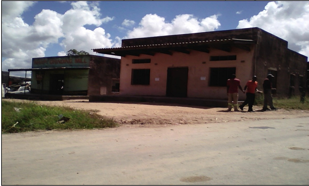
Figure 2: Some of the grinding mills at Murewa growth point
