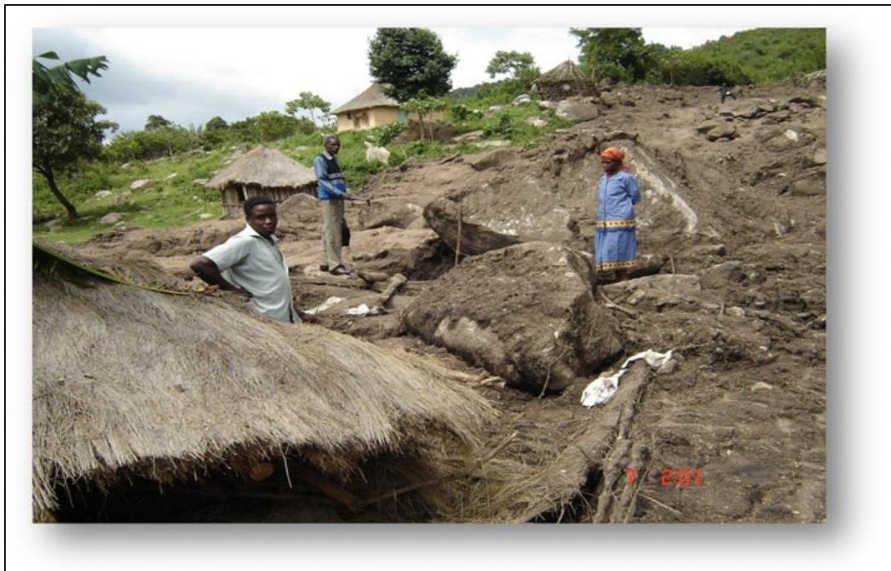
Figure 2: House destroyed by huge rock boulders down a slope due to a landslide.
